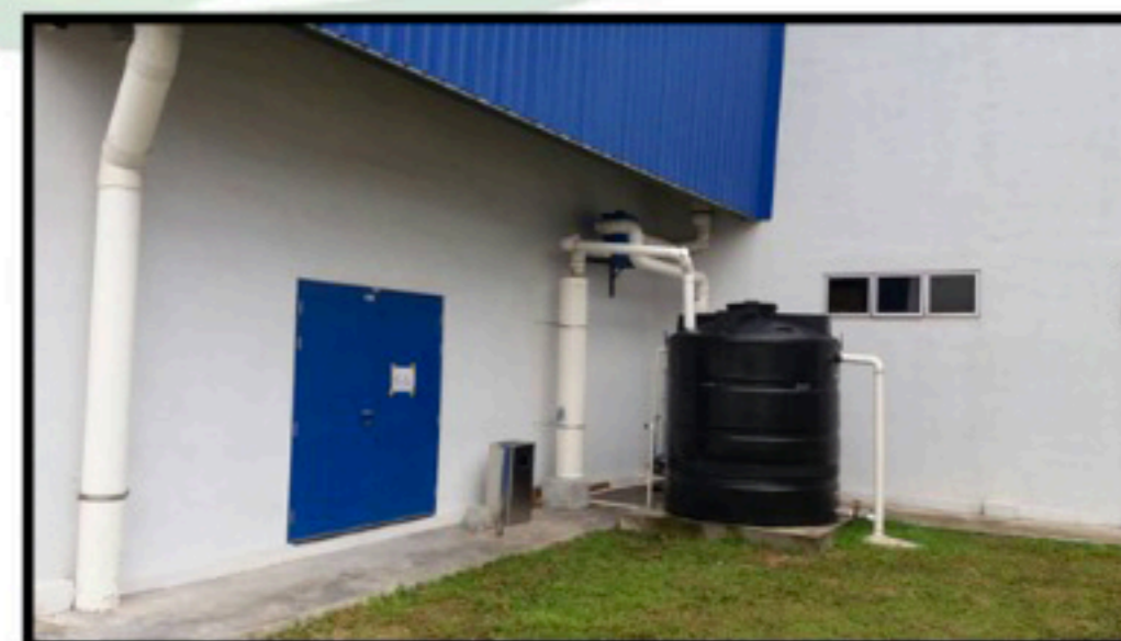
KILANG UMW DEVELOPMENT, SERENDAH
